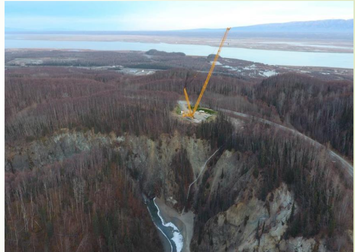
Figure 3-27. View of the construction site (The Conservation Fund, 2017)
