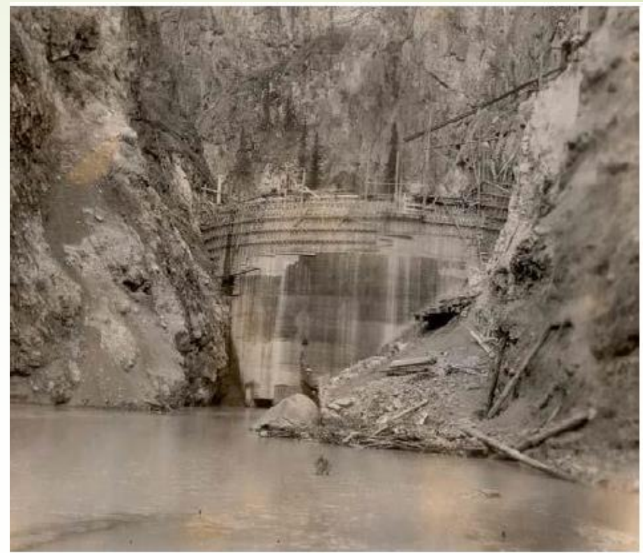
Figure 3-8. Upstream face of diversion dam under construction (CEMML, 2002)
