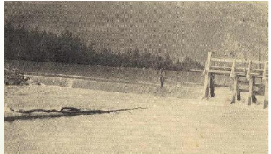
Figure 3-9. Eklutna Lake spillway discharging 1,500 cfs, July 7, 1929 (CEMML, 2002)
