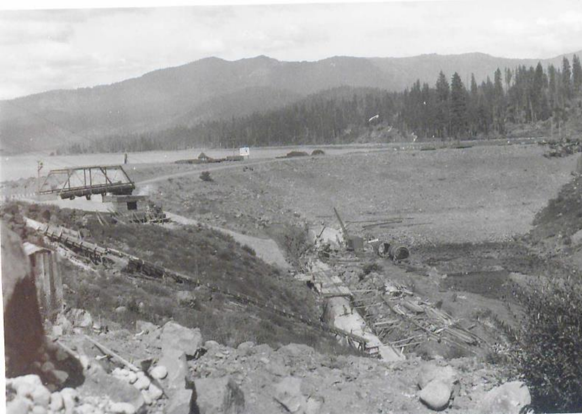
Big Meadows dam construction 1925 (Huber, WRCA)
